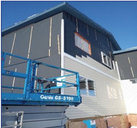
Scammon Bay Teacher Housing Trim Install
